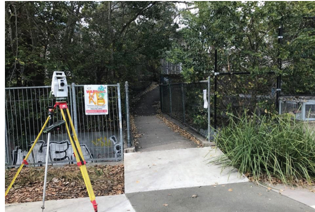
3. An existing concrete bridge over Johnstons Creek connecting pedestrians and cyclists to the Annandale Heritage Conservation area located to west.
